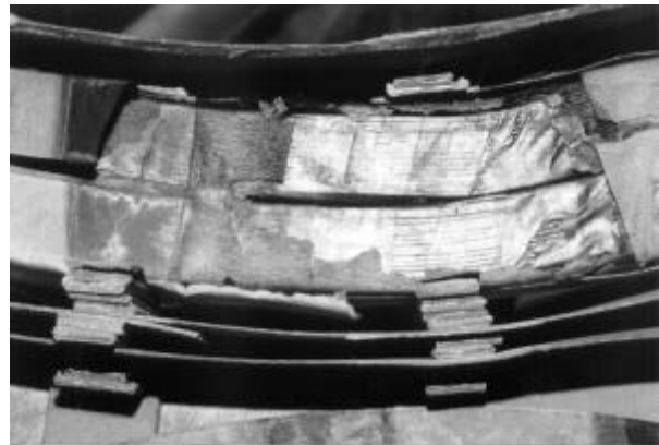
Damage at the bottom of Delta LV winding
